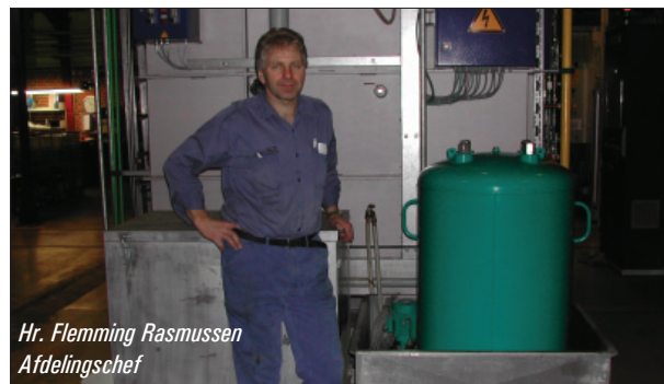
Haustrup Bodycote Installation af CJC™ Finfilter HDU 427/81 MZ
