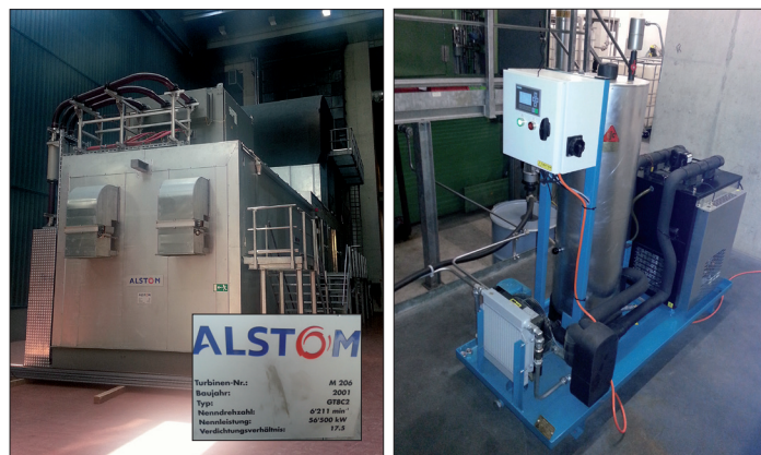
Salzburg AG, Cogeneration Plant, Austria. CJC® Varnish Removal Unit, VRU 27/108 installed at the ALSTOM gas turbine
