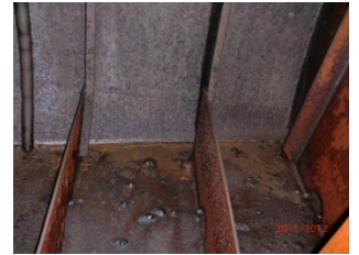
The bottom of a diesel tank, heavy microbial growth
