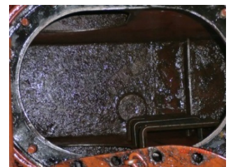
Diesel tank contaminated due to dirt, sludge and water
