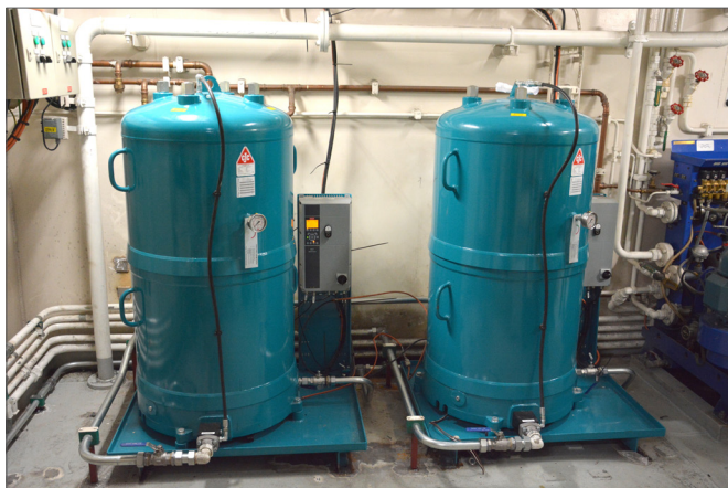
CJC® Engine Lube Oil Filter, 2 x HDU 427/108 installed at Maersk Tracker
