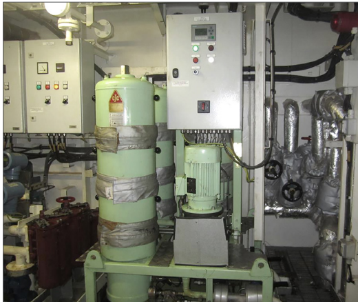
CJC® Marine Diesel Purifier PTU3 3x27/108 Multistay installed at Maersk Involver
