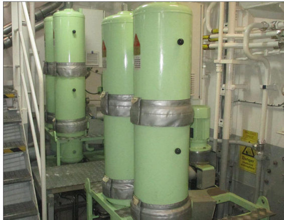
CJC® Marine Diesel Purifier PTU3 2x27/108 Multistay installed at Maersk Mariner
