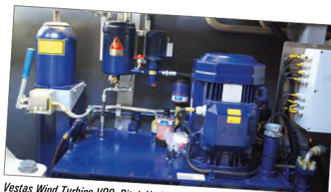
Vestas Wind Turbine V90, Pitch Hydraulic System with a CJC™ HDU 15/25 PV installed
