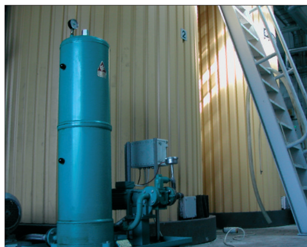
For depth filtering of heat transfer oil plants, a new type CJC™ Fine Filter is developed, which can resist the high pressure in the system. The model is an HP 27/108 and is presently in operation at Daloon, filtering two huge boilers, each containing approx. 7,000 litres of heat transfer oil.
