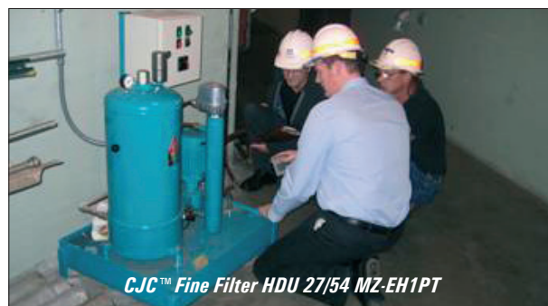
Varnish Removal from Governor System
