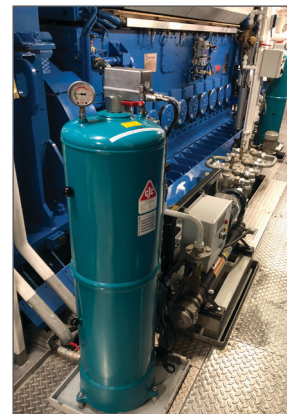
CJC® Fine Filter HDU 27/108 for cleaning of the lube oil
