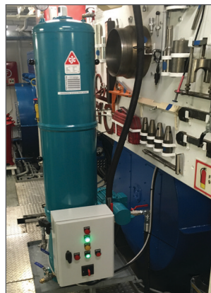
CJC® Filter Separator PTU 27/108 for cleaning of the diesel fuel
